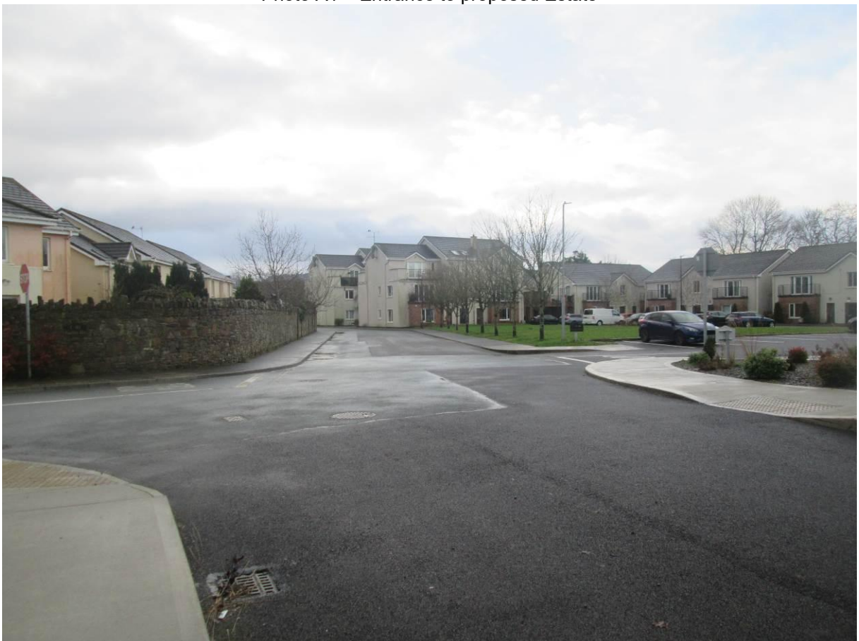
Photo A2 – Access road through exiting residential development to proposed subject site
