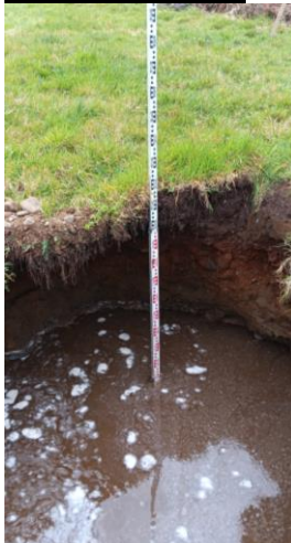
Photo 23 – Trial Hole T5; Water Fill: Level of effective depth at proposed invert (100% level of fill). (2.0m deep) Water level = 1.1m deep. (dimensions 1.5m wide x 1.8m long)
