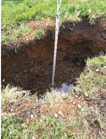
Photo 22 – Trial Hole T4; Water Fill: Level of effective depth at proposed invert (25% level of fill). Water level = 0.275m deep. (dimensions 1.0m wide x 2.0m long)
