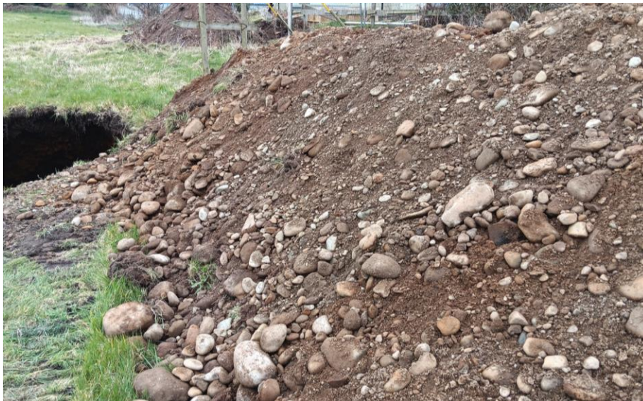
Photo 27 – Trial Hole T1; Spoil from excavation: heterogenous soil: sandy gravel with minor silt content. Some sporadic cobbles (<200mm). No boulders present.
