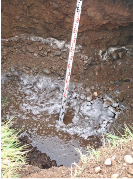
Photo 12 – Trial Hole T2; Water Fill: Level of effective depth at proposed invert (50% level of fill). Water level = 0.550m deep. (dimensions 1.2m wide x 1.6m long)
