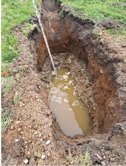
Photo 18 – Trial Hole T3; Water Fill: Level of effective depth at proposed invert (25% level of fill). Water level = 0.350m deep. (dimensions 1.0m wide x 2.0m long)
