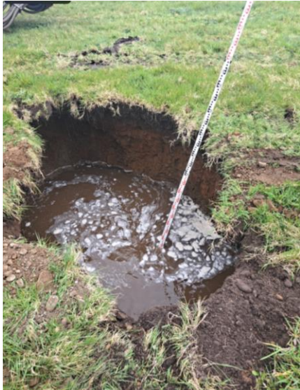
Photo 10 – Trial Hole T2; Water Fill: Level of effective depth at proposed invert (100% level of fill). Water level = 1.1m deep. (dimensions 1.2m wide x 1.6m long)
