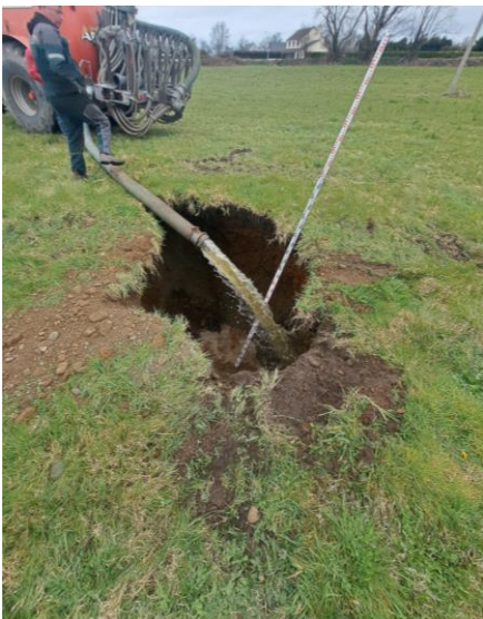
Photo 9 – Trial Hole T2 – during water fill process. (2.4m deep)
