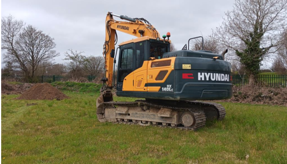
Photo No 2 – Excavator (Hyundai HX 140Lc). Excavated spoil from Trial Hole T5.
