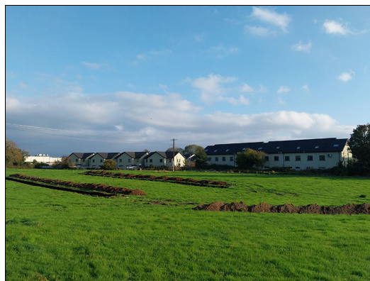
Plate 47. Trenching in progress, from NW, from E.
