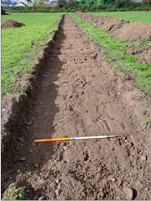
Plate 9. Trench 3, from E.
