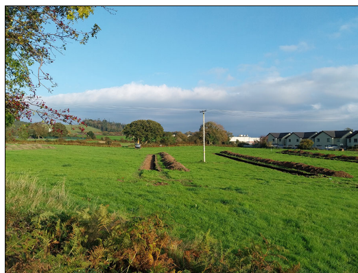
Plate 46. Trenching in progress, from NW, from E.
