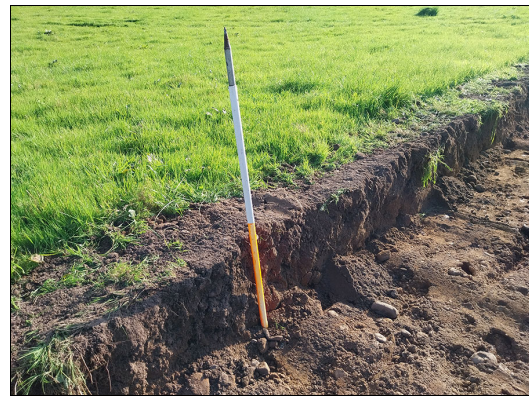
Plate 20. Trench 7, NW facing section, from N.
